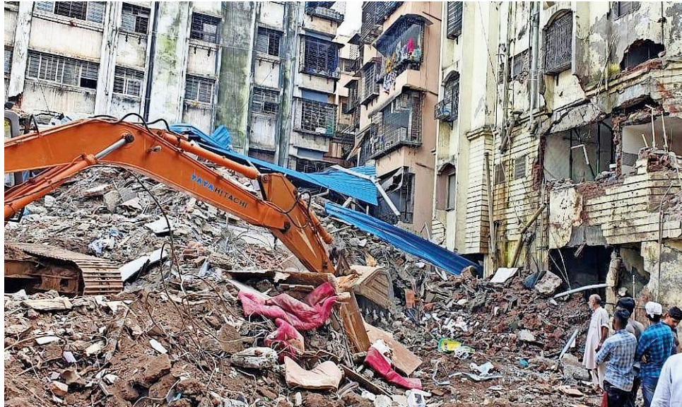
Demolitions of dilapidated buildings being carried out in Ulhasnagar
